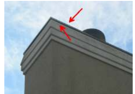
Check cap for leaks real fasteners and gaps as necessary.
