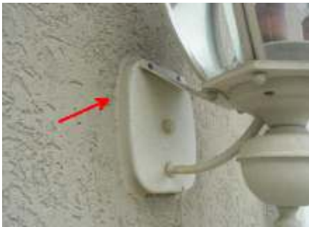
Remove and replace attachments or fixture sealants.
