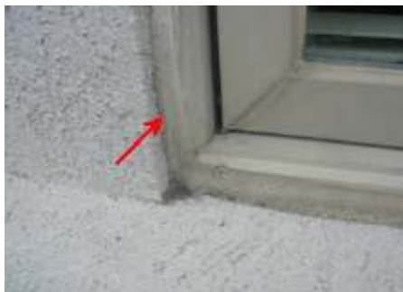
Remove and replace window perimeter sealants.
