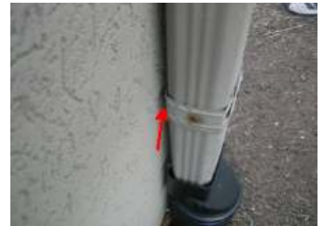
Seal all downspout fasteners.
