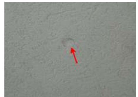
Repair all impact damage.
