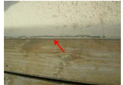
Crack in balcony sealants. No evidence of wall flashing.
