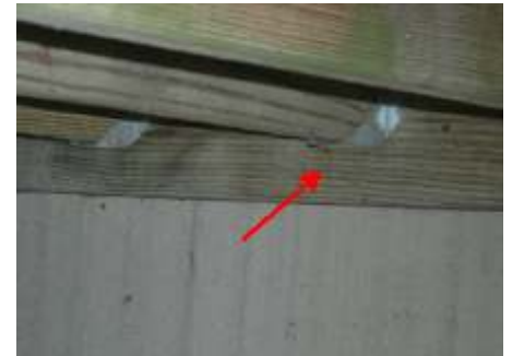
Deck is attached to the eifs. No evidence of flashing.
