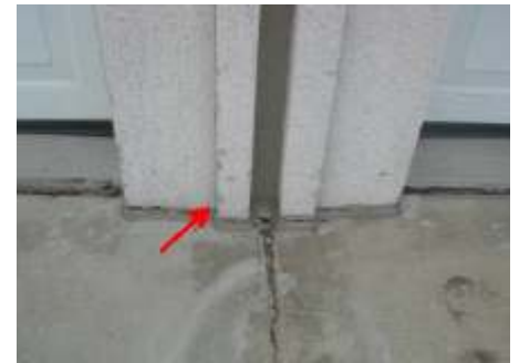
Cut up and repair door trim terminations.
