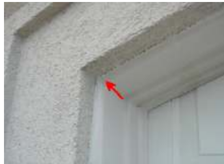
Remove and replace door perimeter sealants.
