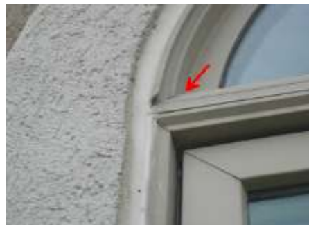
Suggest sealing all window construction joints.
