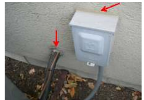
Remove and replace sealants at all utilities.
