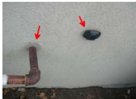
Remove and replace sealants at all siding penetrations.
