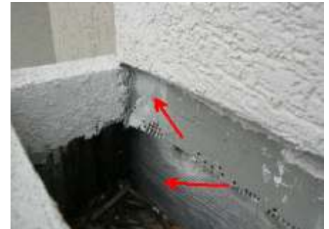
Planter boxes are improperly installed and need to be removed or corrected.
