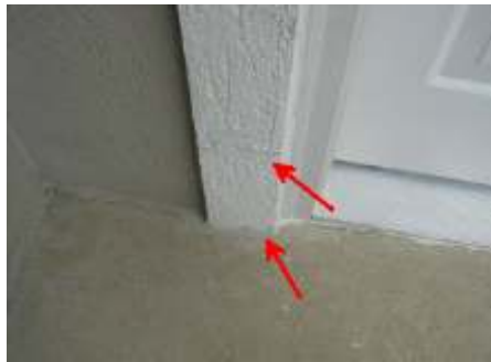
Repair cracking and correct termination at rear garage door.
