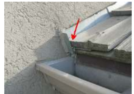
Install new flashing to meet manufacturer specifications.
