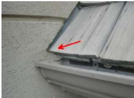
Missing flashing. Install proper kickout flashing.
