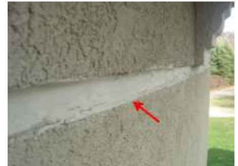
Expansion joint sealants need to be removed and replaced.
