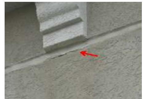
Failing expansion joint sealants under planter boxes.
