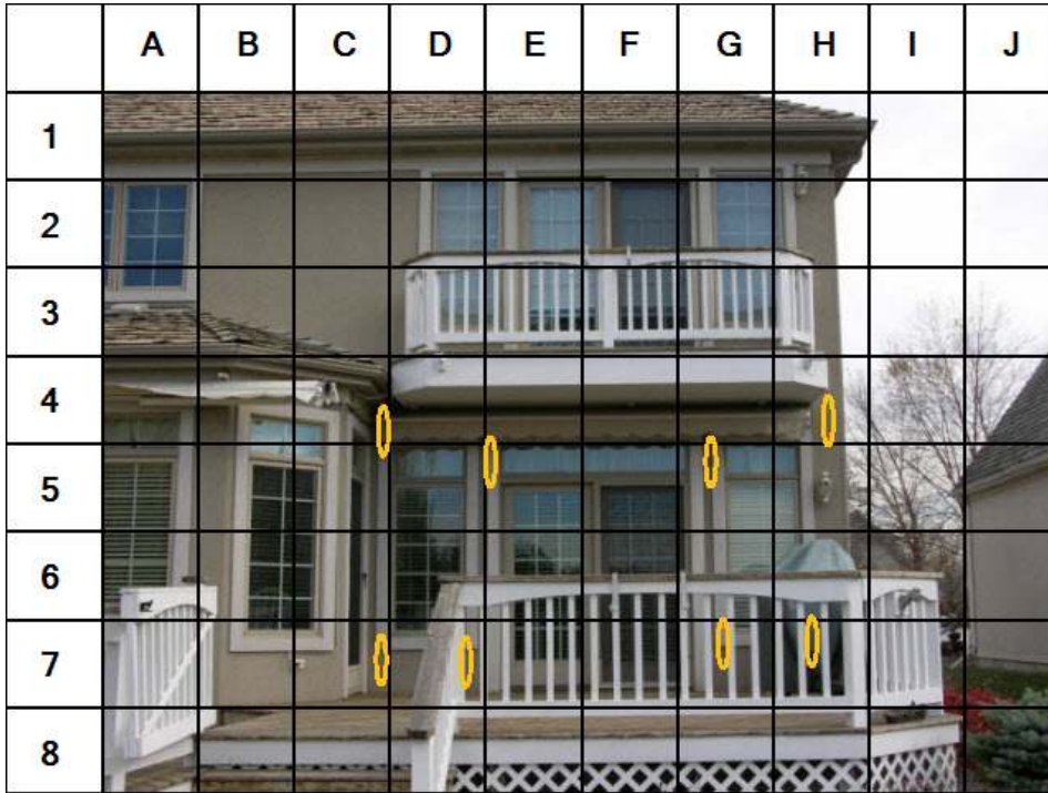
Crack in balcony sealants. No evidence of wall flashing.
